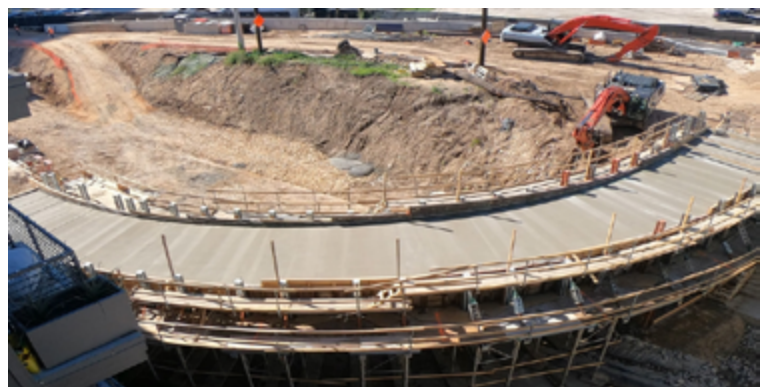
Time-lapse sequence of the concrete pour for the Cypress Grove Bridge. The pour was accomplished in a single overnight effort on October 31. This bridge will connect the creek-level trail to street level at 4th and Sabine Streets. View the time-lapse video here , courtesy of Jay-Reese Contractors.
