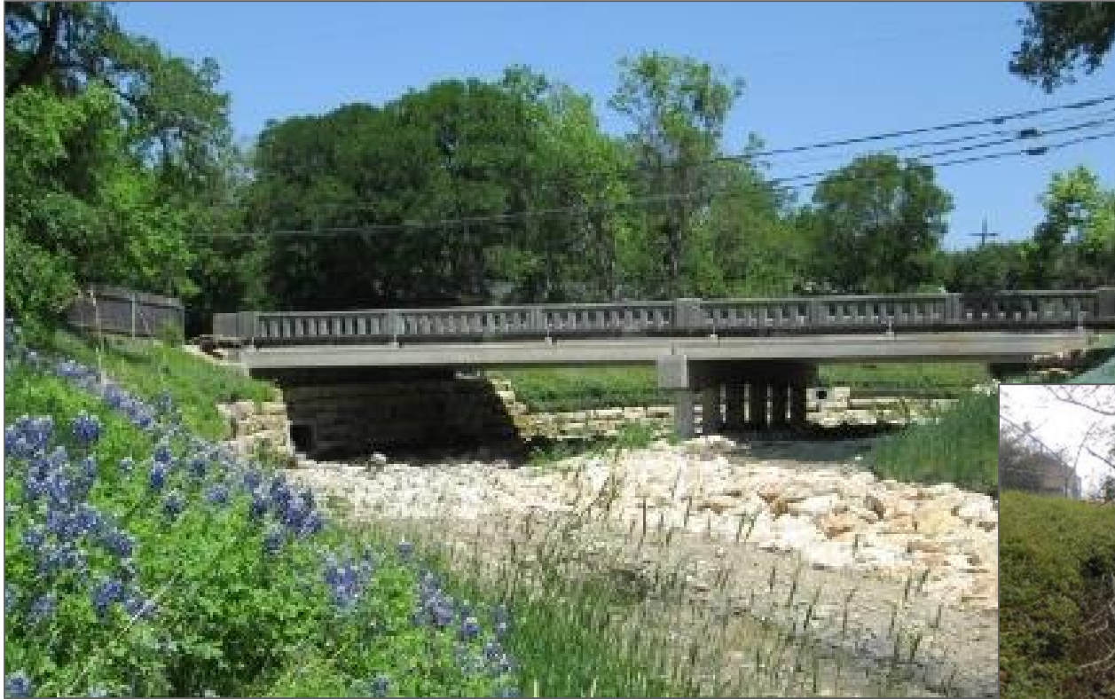
Example project – similar type but longer bridge
