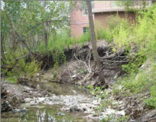
Example project - before
