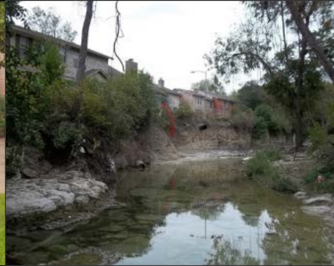
reduce hazards of Erosion
