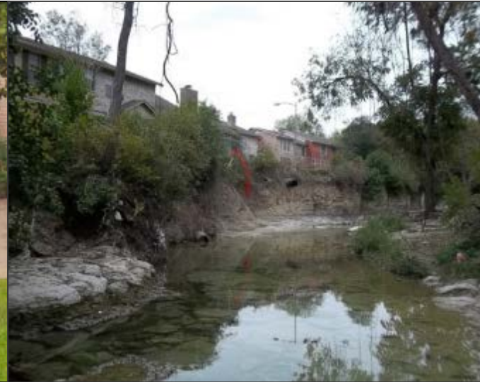
reduce hazards of Erosion
