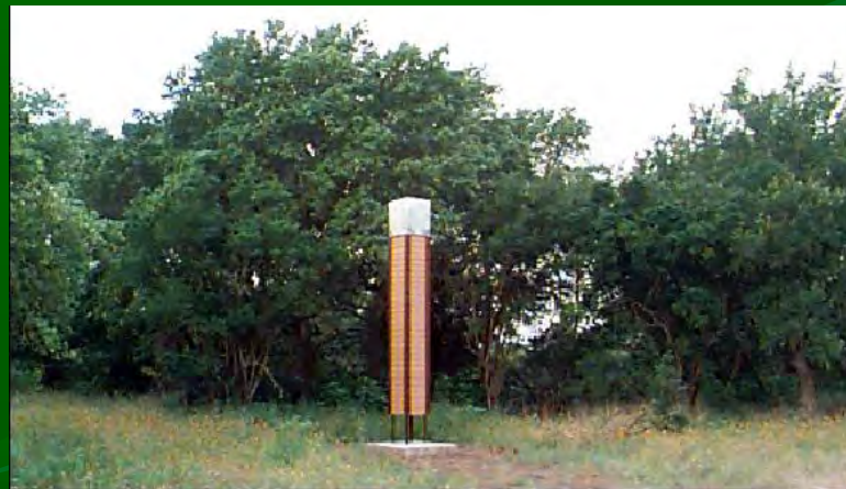
Chimney Swift Tower
