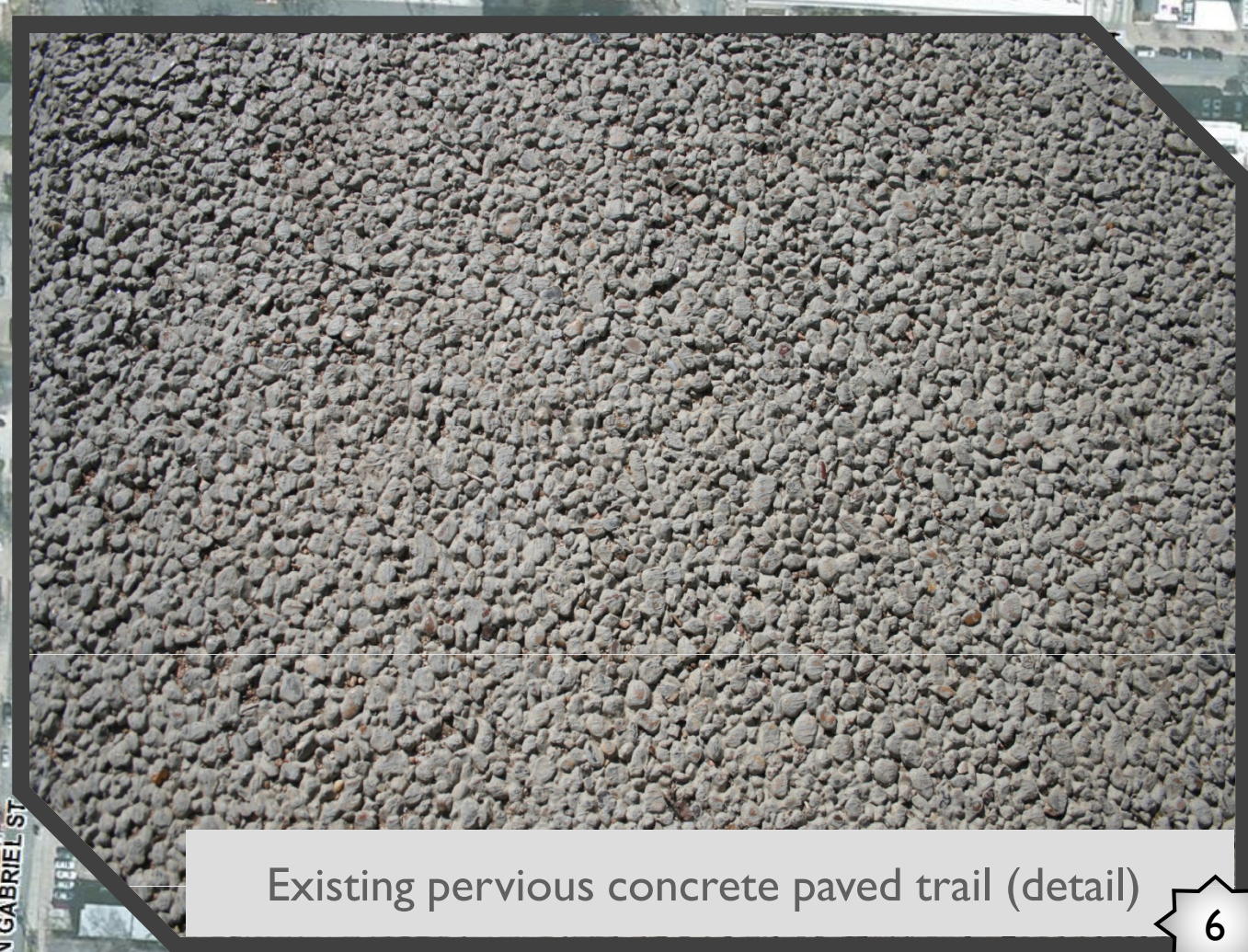
Existing pervious concrete paved trail
