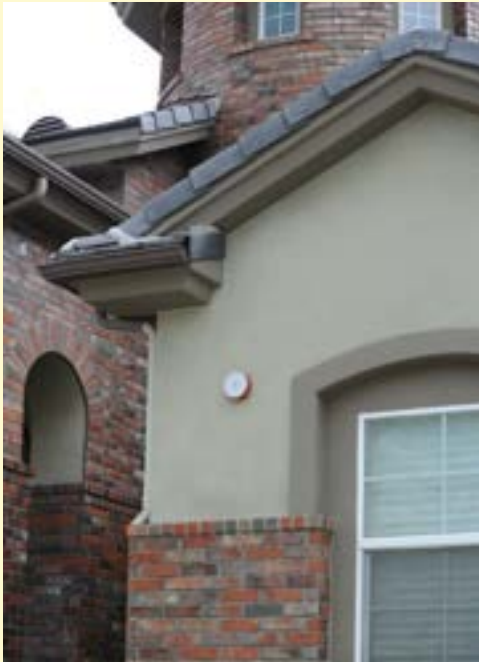
Falling embers from a wildfire can easily ignite leaves and dry debris collected in rain gutters.
