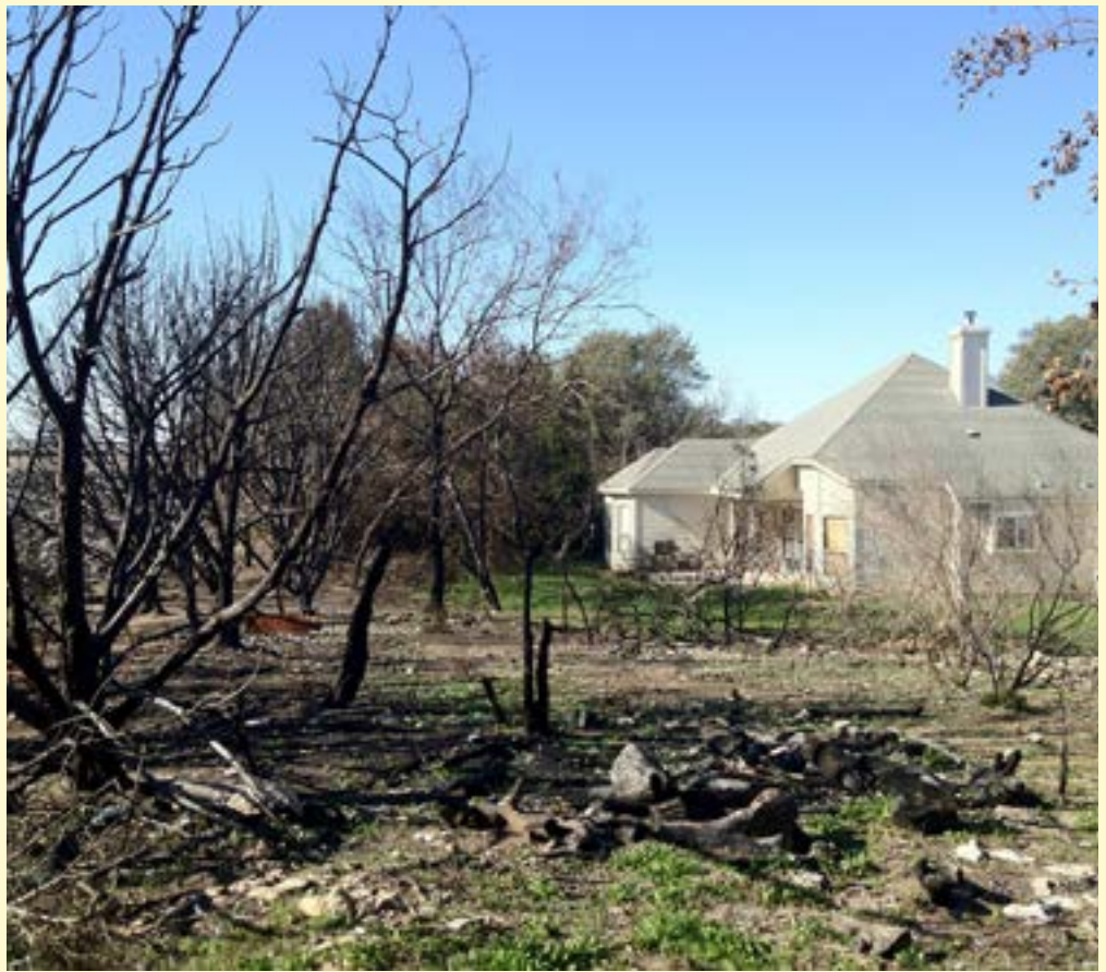
Effective defensible space helped save this home during the Steiner Ranch wildfire in September 2011.
