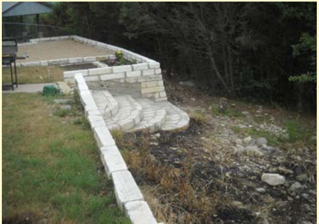
A retaining wall constructed with noncombustible materials can help prevent a fire from moving up a slope, and provides key defense to homes located on steep topography.
