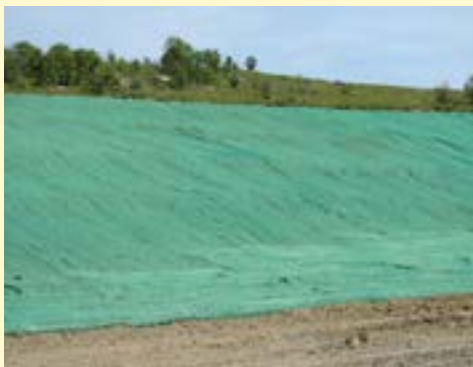
Erosion control blankets
