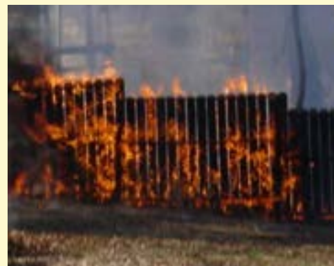
Wooden privacy fences can act as a wick and carry fire directly to your home.
