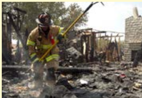
Ash from chemically-treated building materials, such as pressure treated lumber, can be toxic and require special disposal.
