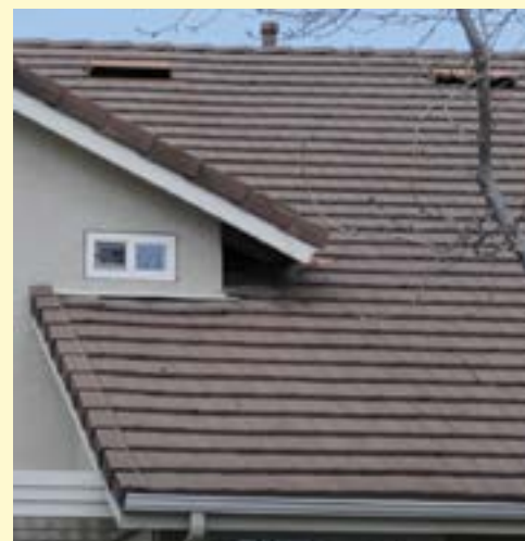
Use ignition-resistant, Class A-rated roofing materials and keep roof surfaces clear of debris.
