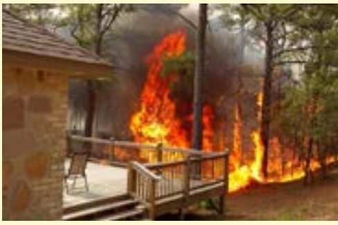
This Bastrop home had an attached wooden deck surrounded by dense vegetation. These types of conditions often result in home loss during a wildfire event.
