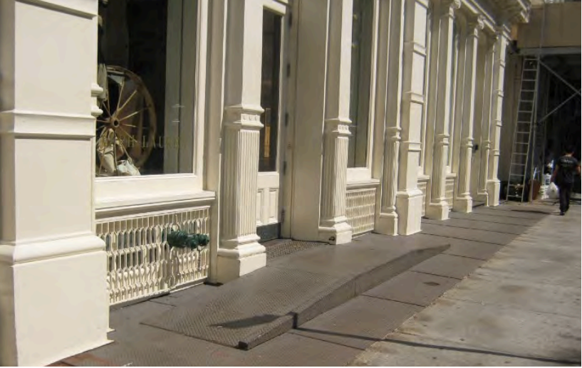
Above: Ramps and chair lifts can provide access while preserving historic character.
