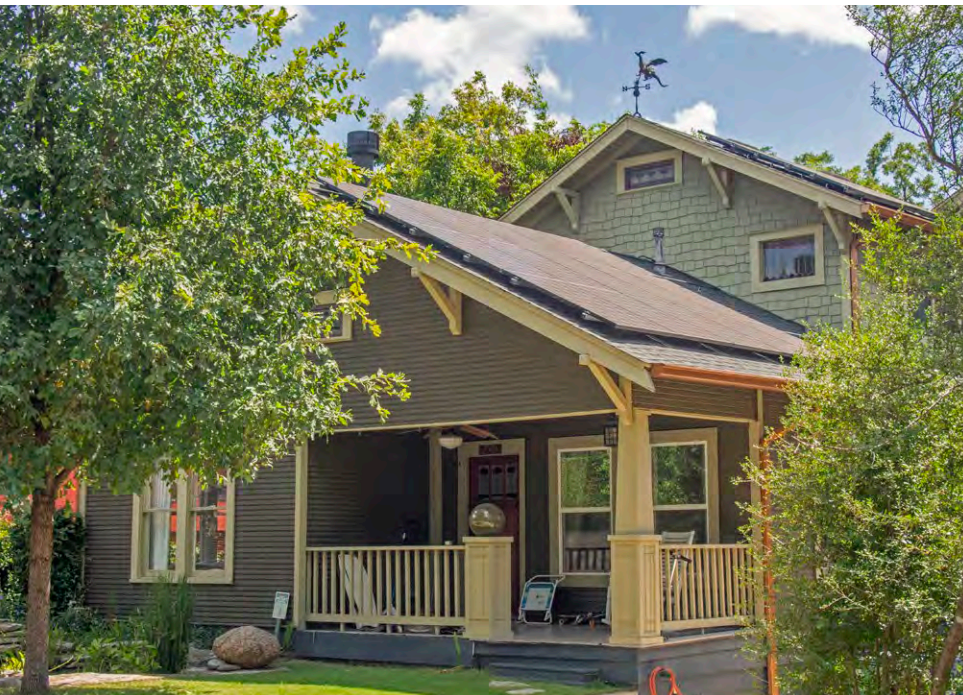
For additions to buildings with front-gabled, flat, or shed roofs, if the front wall is thirty feet (30') wide, set the addition back by at least fifteen feet (15').
