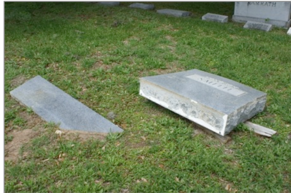
Epoxy appears to have been applied only around the perimeter of headstones in Austin Memorial Park Cemetery: (left) in Section 5; (right) in Section 1
