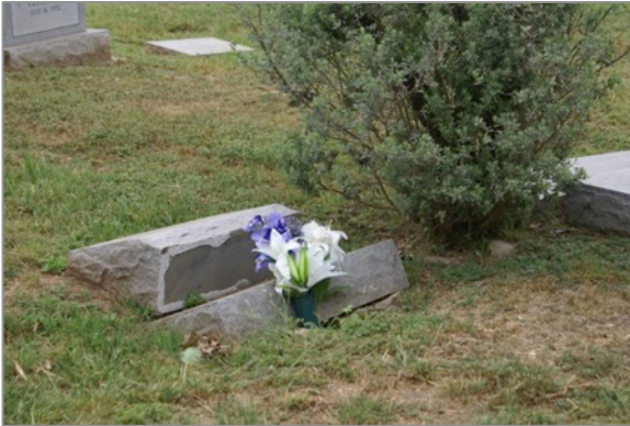
Epoxy appears to have been applied only around the perimeter of headstones in Austin Memorial Park Cemetery: (left) in Section 5; (right) in Section 1
