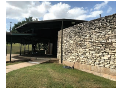
Pool Building - Limestone Wall
