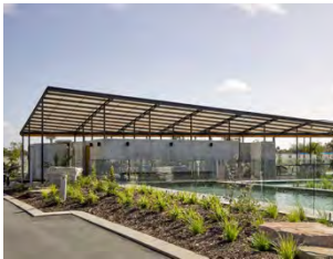
Concrete Walls & Steel Frame 5 votes
