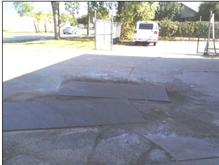
Driveway at Fire Station 24, 5811 Nuckols Crossing
