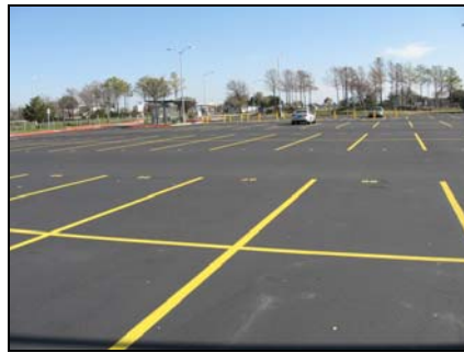
Public Parking Resurfacing
