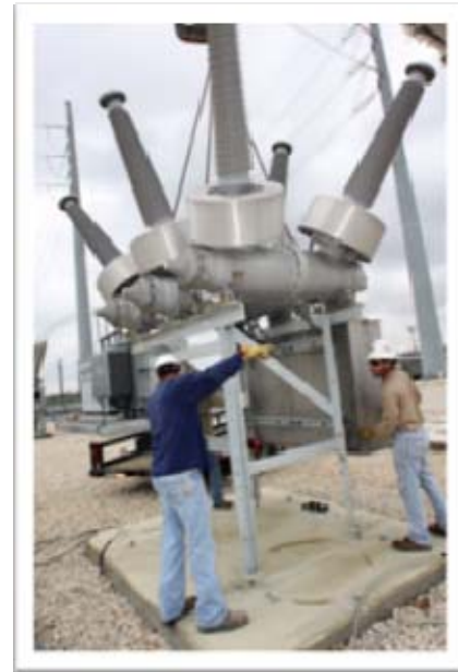
Transformer Installation at the Dessau Substation
