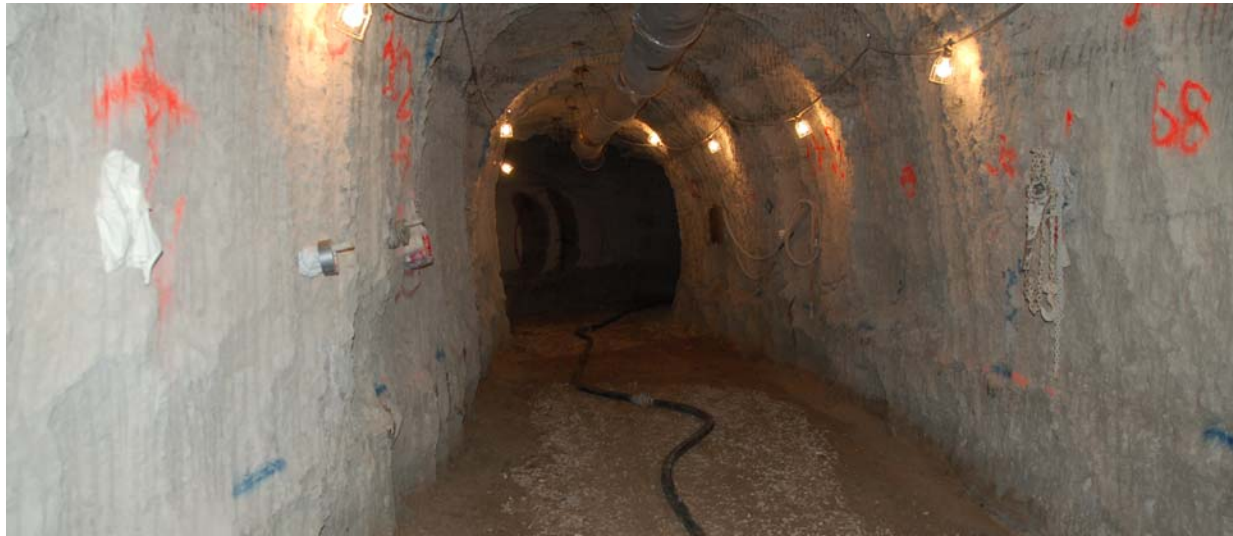
Downtown Wastewater Tunnel
