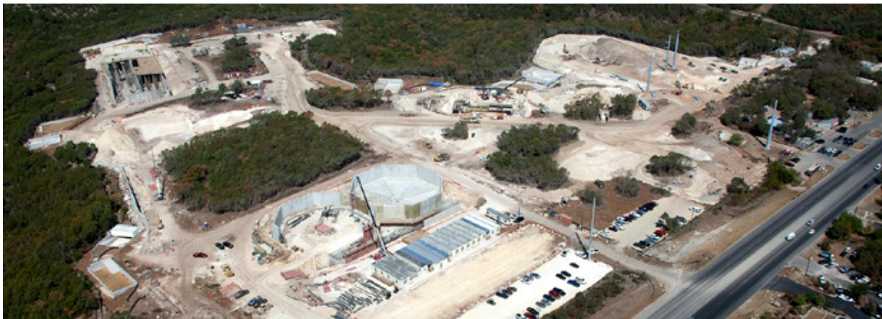
Water Treatment Plant 4 Site at Bullick Hollow
