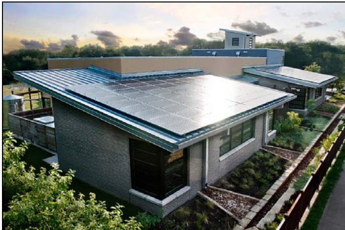
Twin Oaks Branch Library
