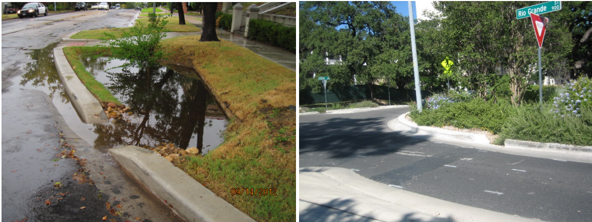
Rain gardens along the Rio Grande Bike Boulevard on 18th and 12th Streets
