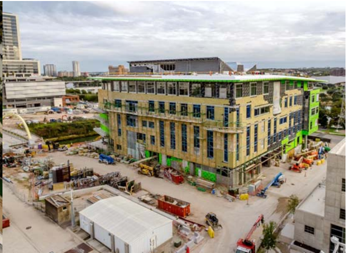
New Central Library – View from West Ave
