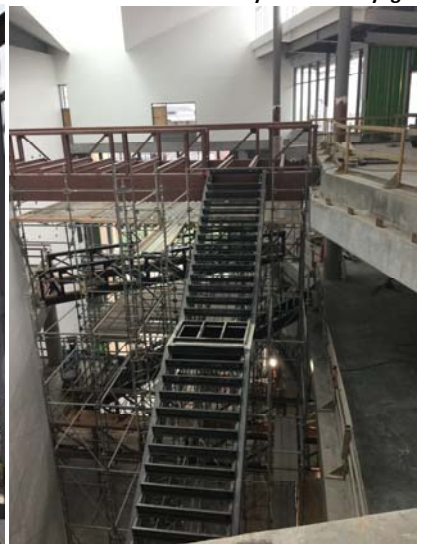
New Central Library – Atrium Stair
