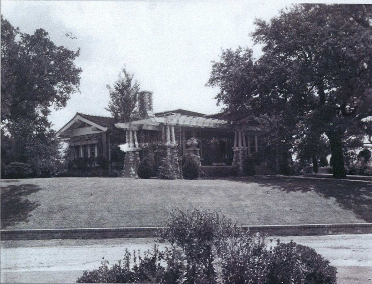
View northeast of the Norwood house from Edgecliff Terrace showing pergola, battered columns with river stone and entry path on far right.
