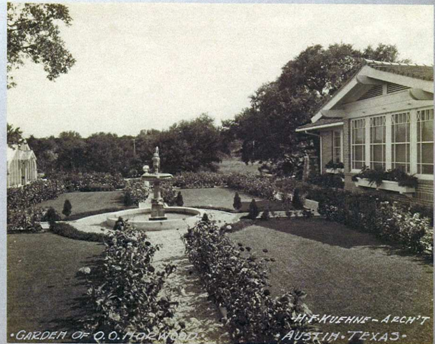
Formal garden walk and fountain and east elevation of house, view south
