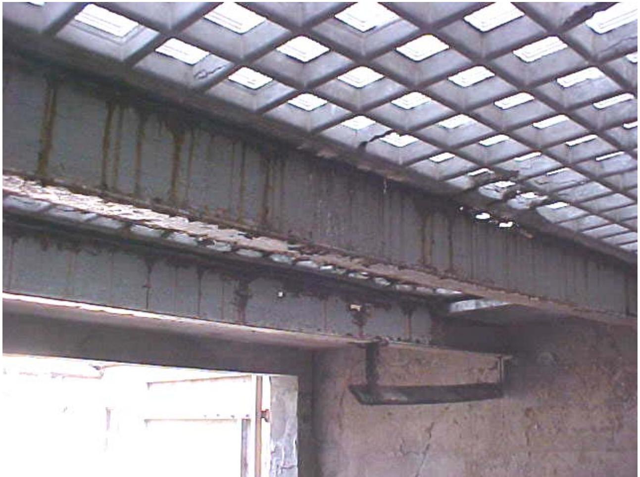
View of underside of glass-brick paving in garage built ca. 1965, showing deterioration of steel beams
