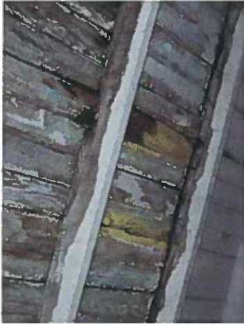
5 FRONT PORCH RAFTERS AND ROOF DECK ROTTED
