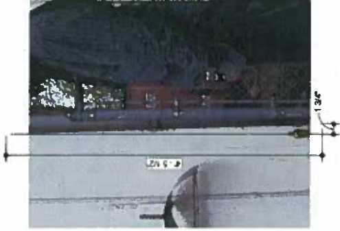
3 NORTHEAST CORNER OUT OF PLUMB
