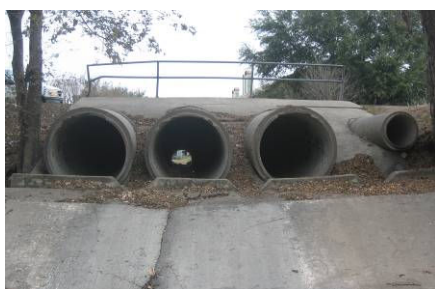
Drainage culverts underneath Masterson Pass
