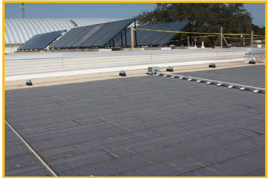
18-kilowatt solar roof & solar hot water system installed at Austin Animal Center (under construction)
