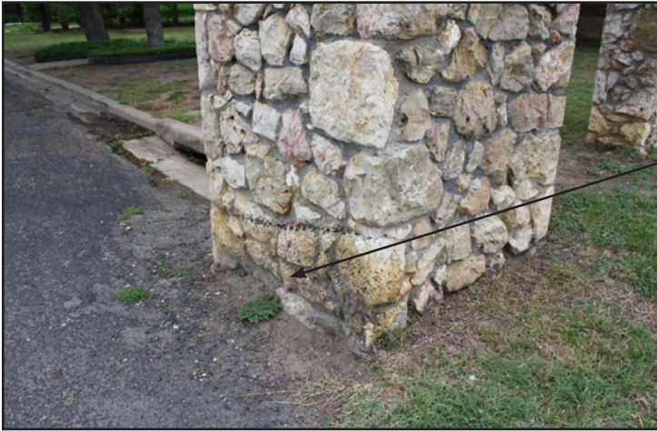
Figure 6: Tar has splashed up from the road on to the entry archway.
