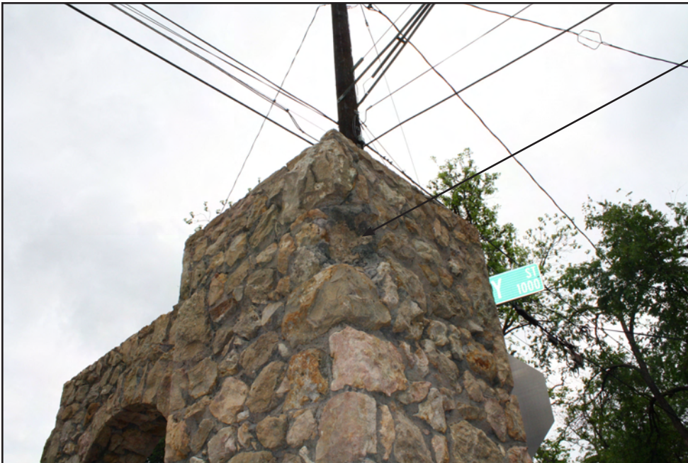
Figure 7: Missing limestone from the entry archway.
