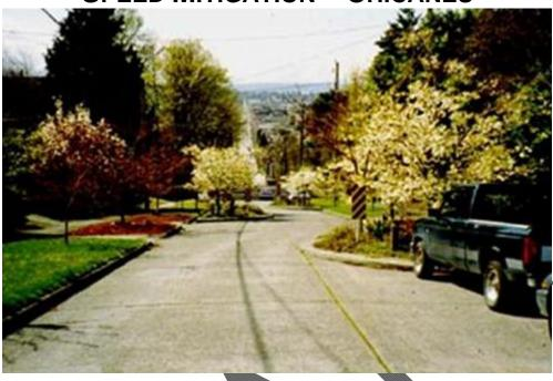
Chicanes are curb extensions that alternate from one side of the street to the other, forming S-shaped curves. Chicanes can also be created by alternating on-street parking, either diagonal or parallel, between one side of the street and the other. Each parking bay can be created either by re-striping the roadway or by installing raised, landscaping islands at the ends of each parking bay.
