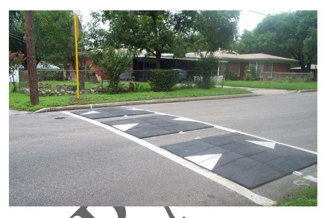
Speed cushions are flat-topped speed humps sections installed across the roadway, with sections of roadway exposed between them; resembling a separated speed hump. They are often constructed with either asphalt or installed using prefabricated rubber cushions. Speed cushions force cars to slow down as they ride with one or both wheels on the humps, but are typically spaced far apart to allow vehicles with wider axles, such as emergency vehicles can straddle them with minimal impact to speed.
