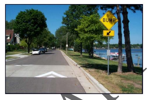
Speed tables are flat-topped speed humps often constructed with brick or other textured materials on the flat section. Speed tables are typically long enough for the entire wheelbase of a passenger car to rest on the flat section. Their long flat fields give speed tables higher design speeds than Speed Humps. The brick or other textured materials improve the appearance of speed tables, draw attention to them, and may enhance safety and speed-reduction.
