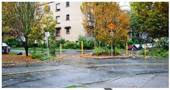
Diagonal diverters are barriers placed diagonally across an intersection, blocking through movements and creating two separate, L-shaped streets. Like half closures, diagonal diverters are often staggered to create circuitous routes through the neighborhood as a whole, discouraging non-local traffic while maintaining access for local residents. They are good for inner-neighborhood locations with non-local traffic volume problems.
