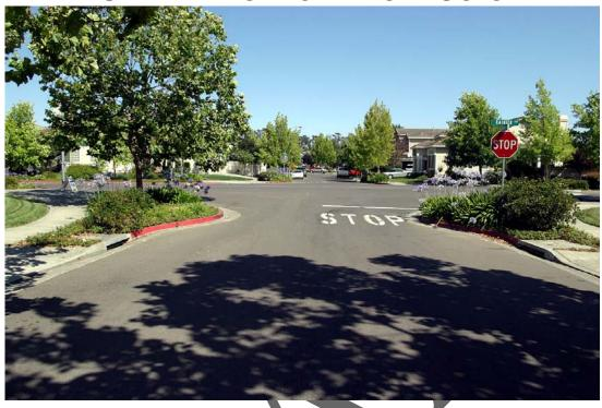
Bulb Outs are curb extensions at intersections that reduce the roadway width from curb to curb. They "pedestrianize" intersections by shortening crossing distances for pedestrians and drawing attention to pedestrians via raised peninsulas. They also tighten the curb radii at the corners, reducing the speeds of turning vehicles.
