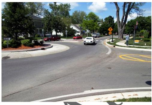
Roundabouts are raised landscaped islands that require traffic to circulate counterclockwise around a center island. Roundabouts are used on higher volume streets to allocate right-of-way between competing movements.
