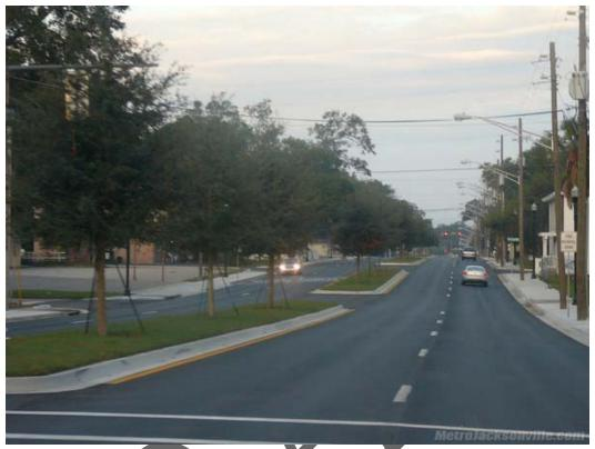
Median barriers are islands located along the centerline of a street and continuing through an intersection so as to block through movement at a cross street.
