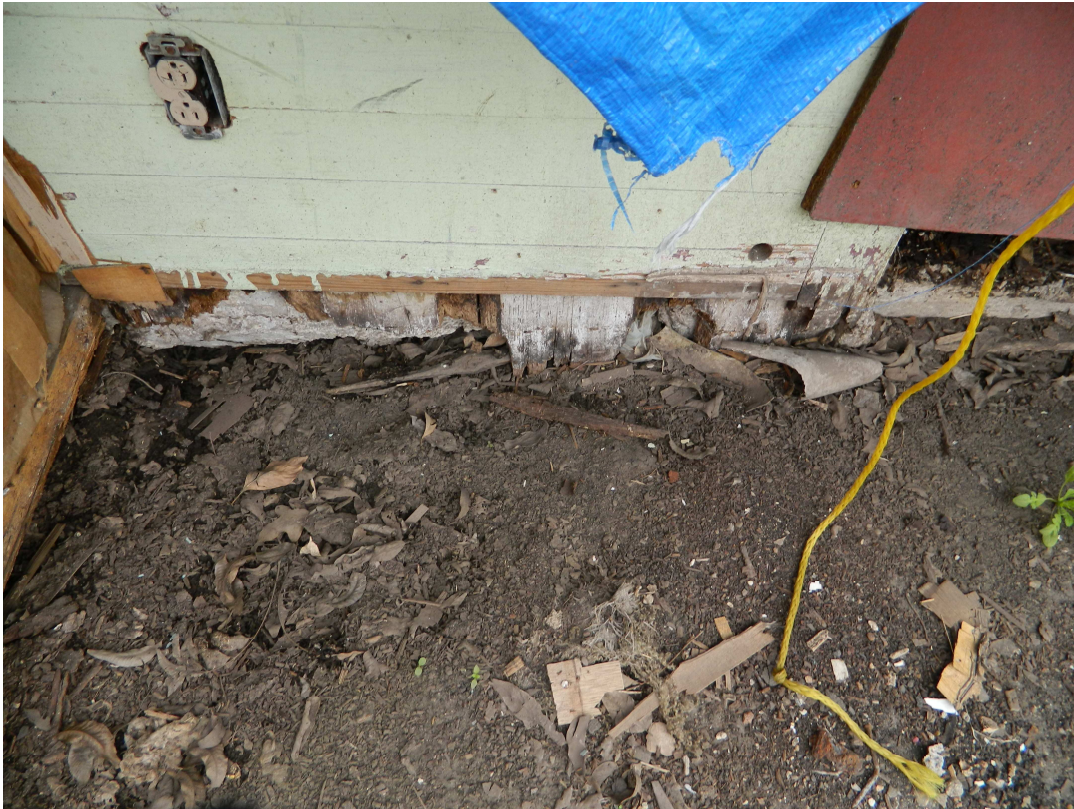
Detail view of the boards (missing battens) at the sill; south side of the building. The interior wall of the now-demolished rear addition covers the original boards.
