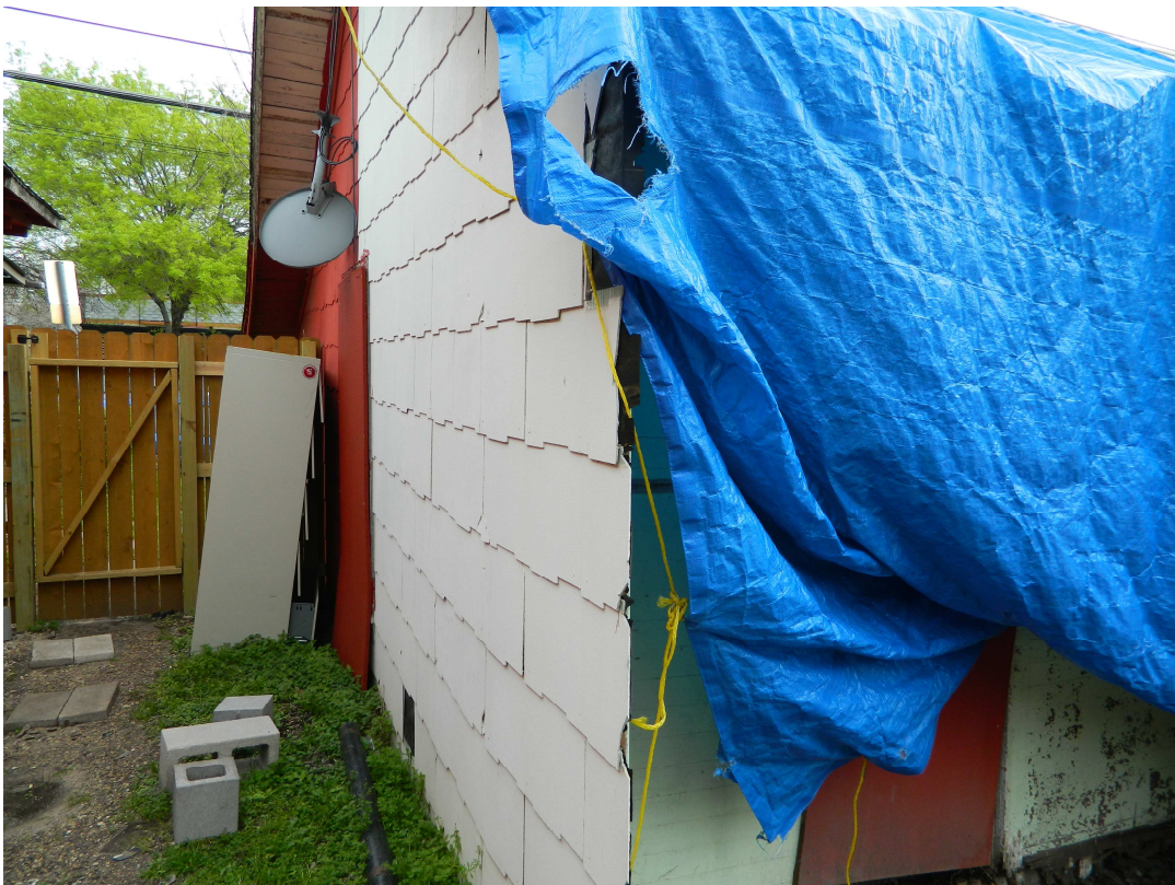
The west side of the building has asbestos siding; a horizontally-laid wood wall is underneath.
