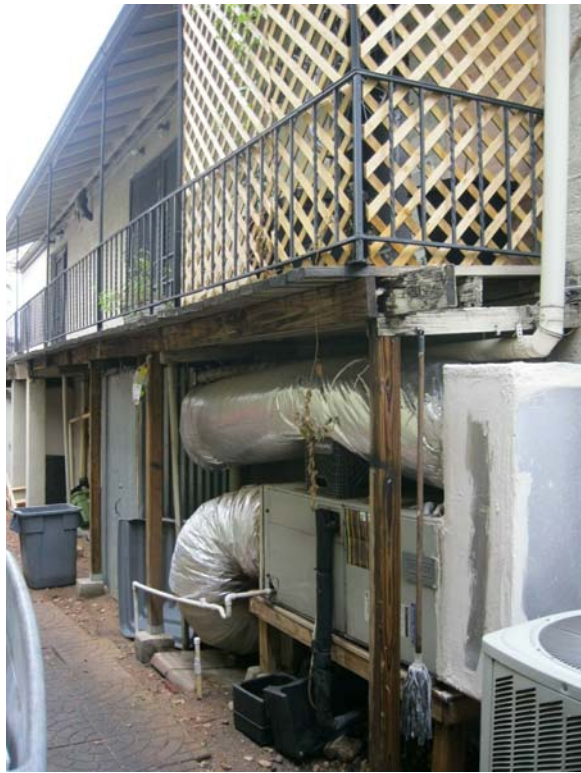
JEFFREY'S - NORTH ELEVATION - HVAC EQMT & WOOD BALCONY TO BE REMOVED.
