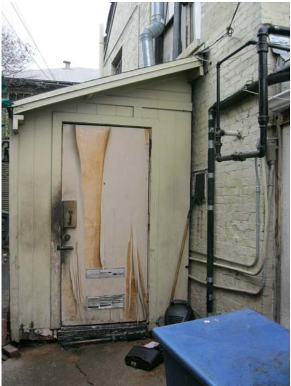
JEFFREY'S - WEST ELEVATION - WATER HEATER SHED TO BE REMOVED
