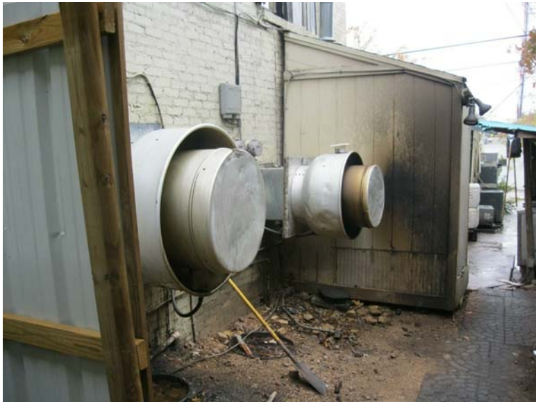
JEFFREY'S - WEST ELEVATION - EXHAUST FANS TO BE REMOVED
