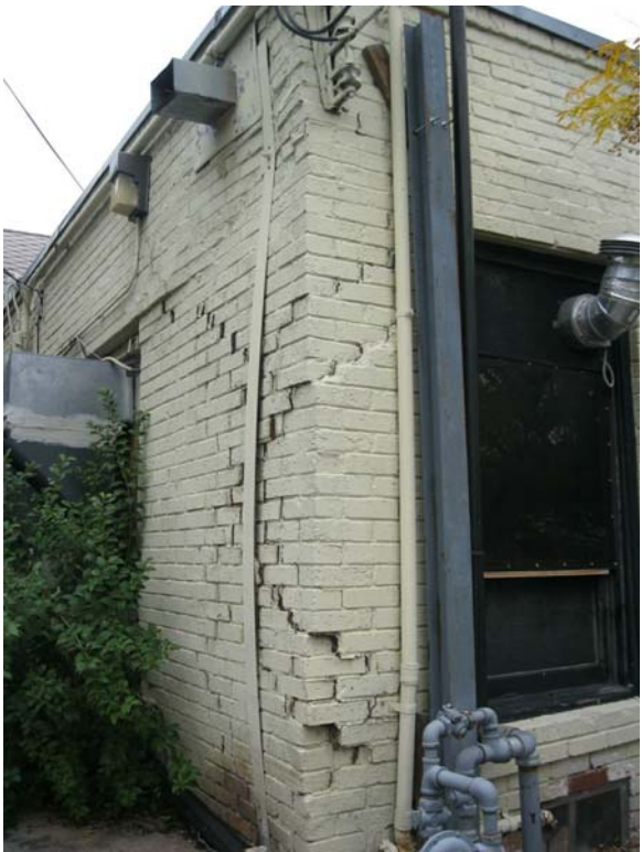
JEFFREY'S - DAMAGED SW CORNER
