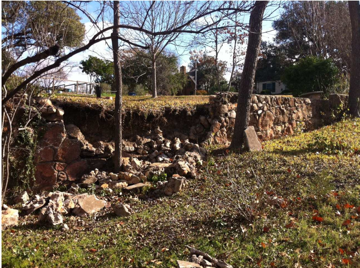
View of the failed section of the stone wall.
