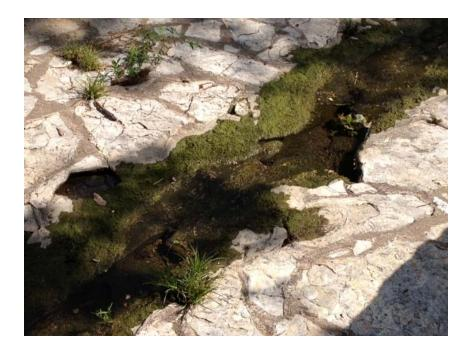
Existing missing parts of the drainage channel bottom, from Wheeler Street to the storm water outlet (approximately 165 linear feet) will be repaired with rock and mortar by this project as mitigation and payment for use of Park land.
