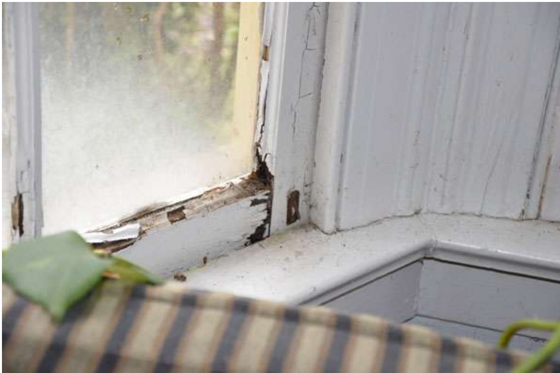
Existing window sash with evidence of wood rot
