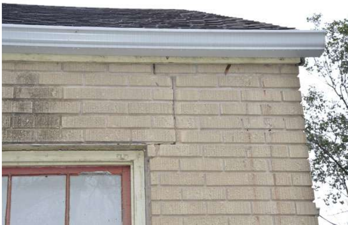
Cracked exterior wall
