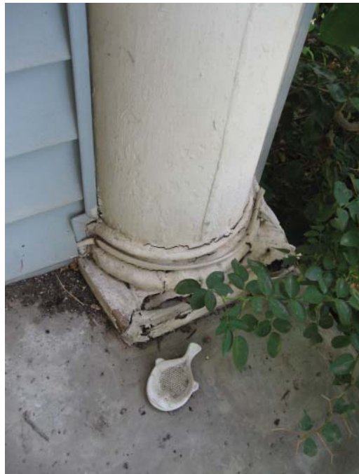
WOOD ROT AT BASE OF EXISTING PILASTERS
