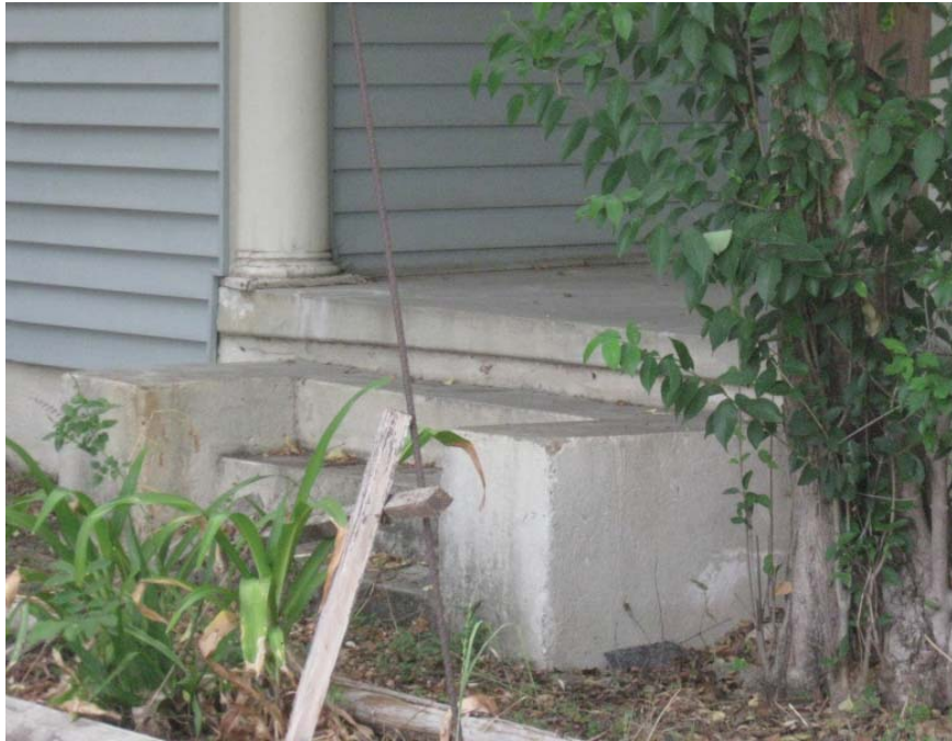
EXISTING STAIR NOT CODE COMPLIANT, TO BE REPLACED
