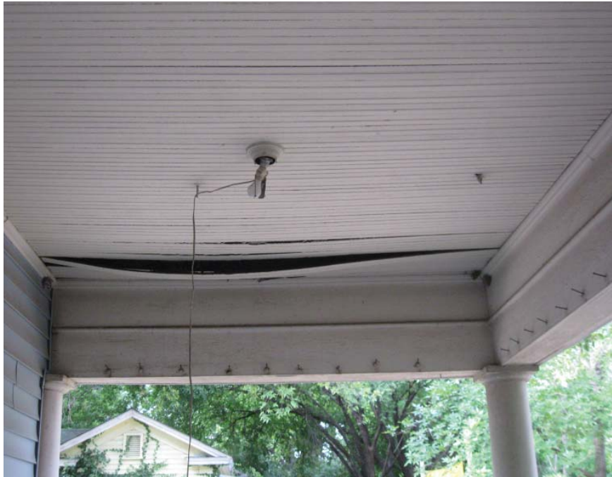
WATER DAMAGE AT CEILING OF EXISTING PORCH
