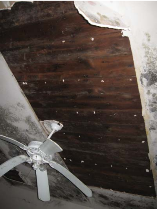
WATER DAMAGE AT INTERIOR CEILING
