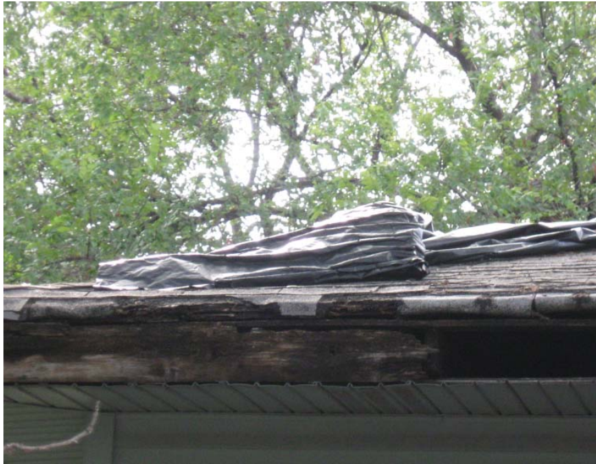
TYPICAL CONDITION AT EXISTING ROOF AND FASCIA
