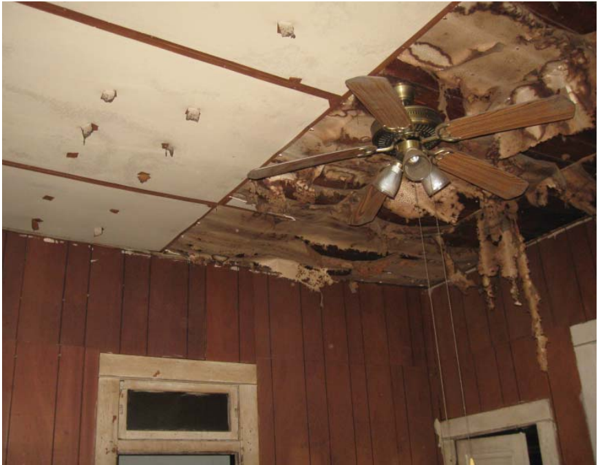
WATER DAMAGE AT INTERIOR CEILING
