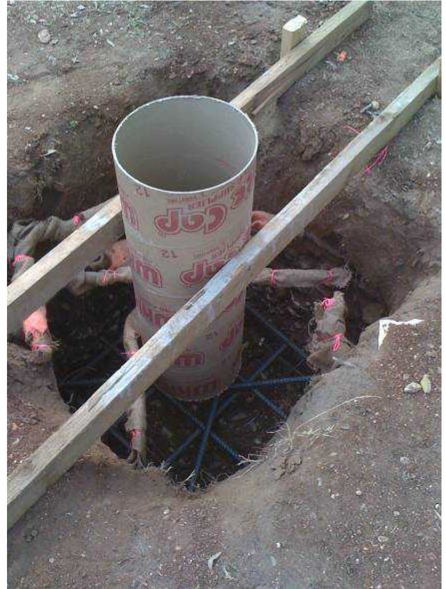
PHASE 1b. Setting steel reinforcing and forms around roots
