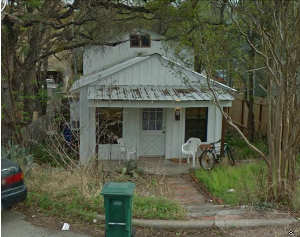
Front elevation of 1612 W. 11th Street
