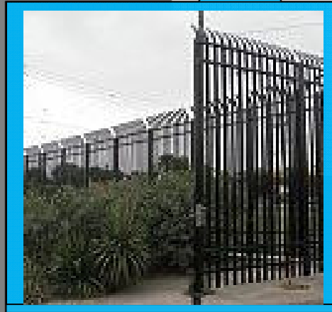
Proposed Steel Picket South Woods Only Height - 8' ht.
