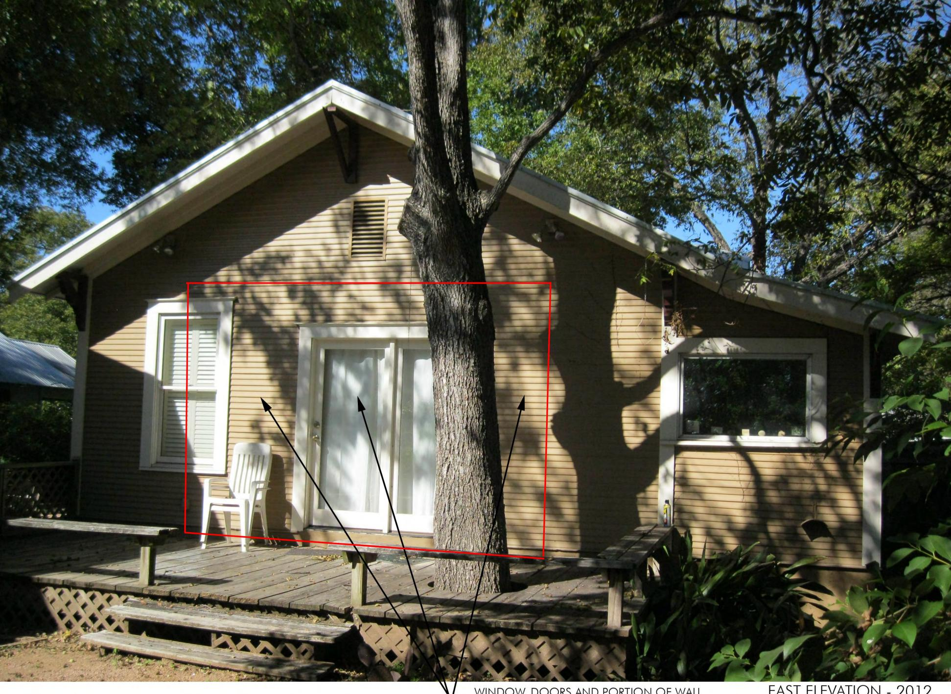
WINDOW, DOORS AND PORTION OF WALL TO BE DEMOLISHED
