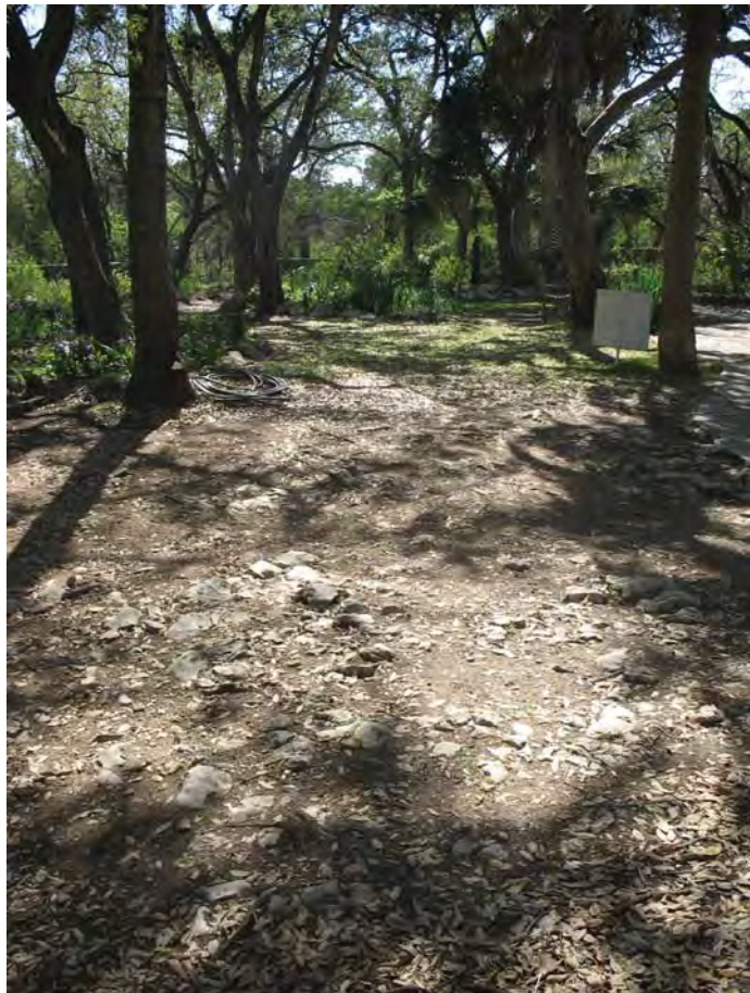
View facing West from Arch: erosion exposing stones and rock subgrade
