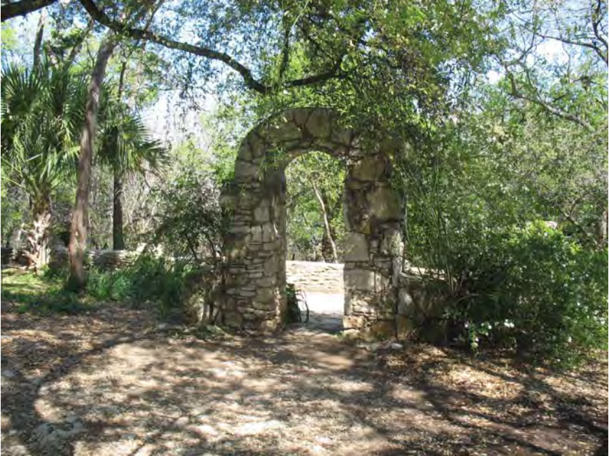
View facing East toward Arch-- erosion exposing stones and depositing soil into archway/overlook area
