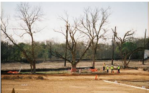
Figure 37: Examples of tree preservation during construction.
