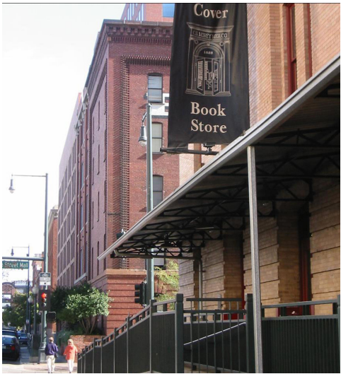
Figure 38: Example of an ADA ramp with shade structure.
