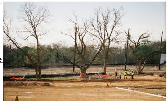
Figure 37: Examples of tree preservation during construction.
