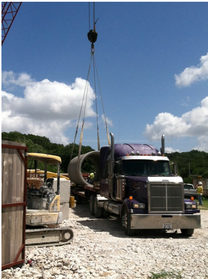
Pipe Delivery at Spicewood Shaft
