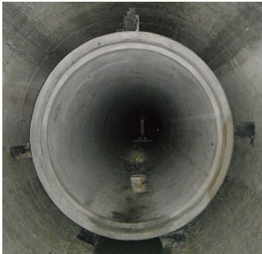
Pipe placement in tunnel
