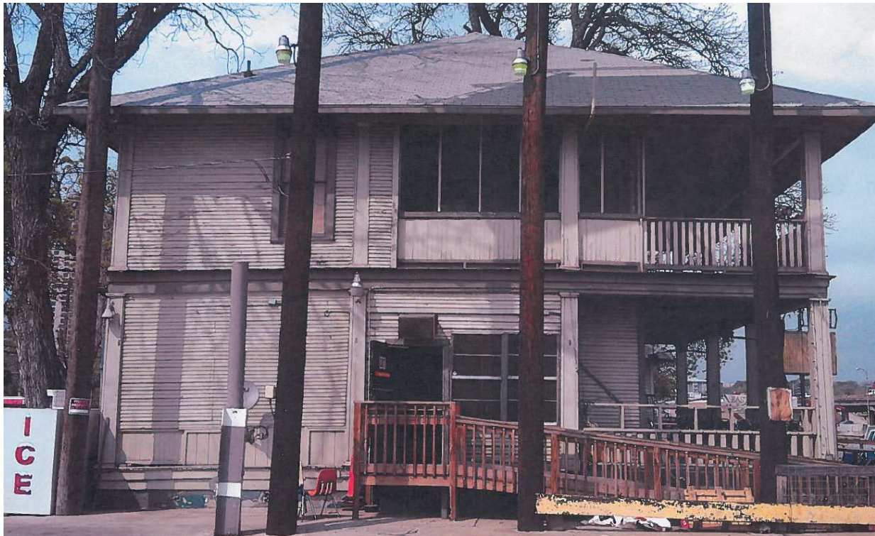
South elevation, showing the portions of the historic wraparound porch that have been enclosed.
