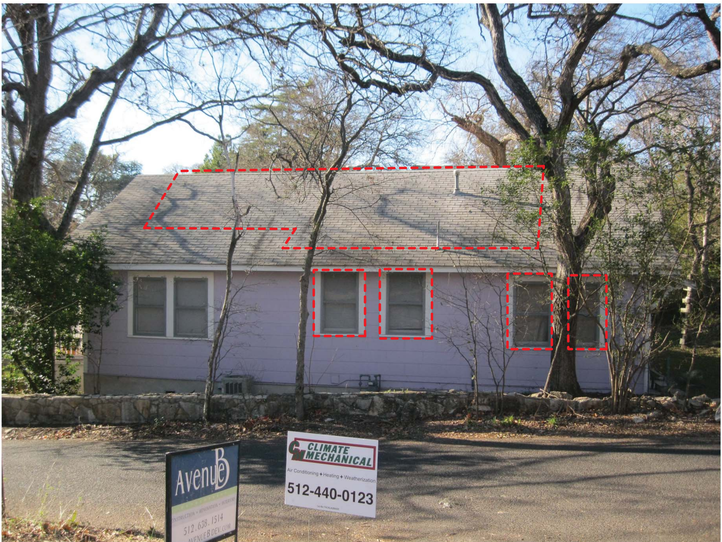
DEMOLITION OF PORTION OF ROOF; REMOVAL OF EXISING WINDOWS
