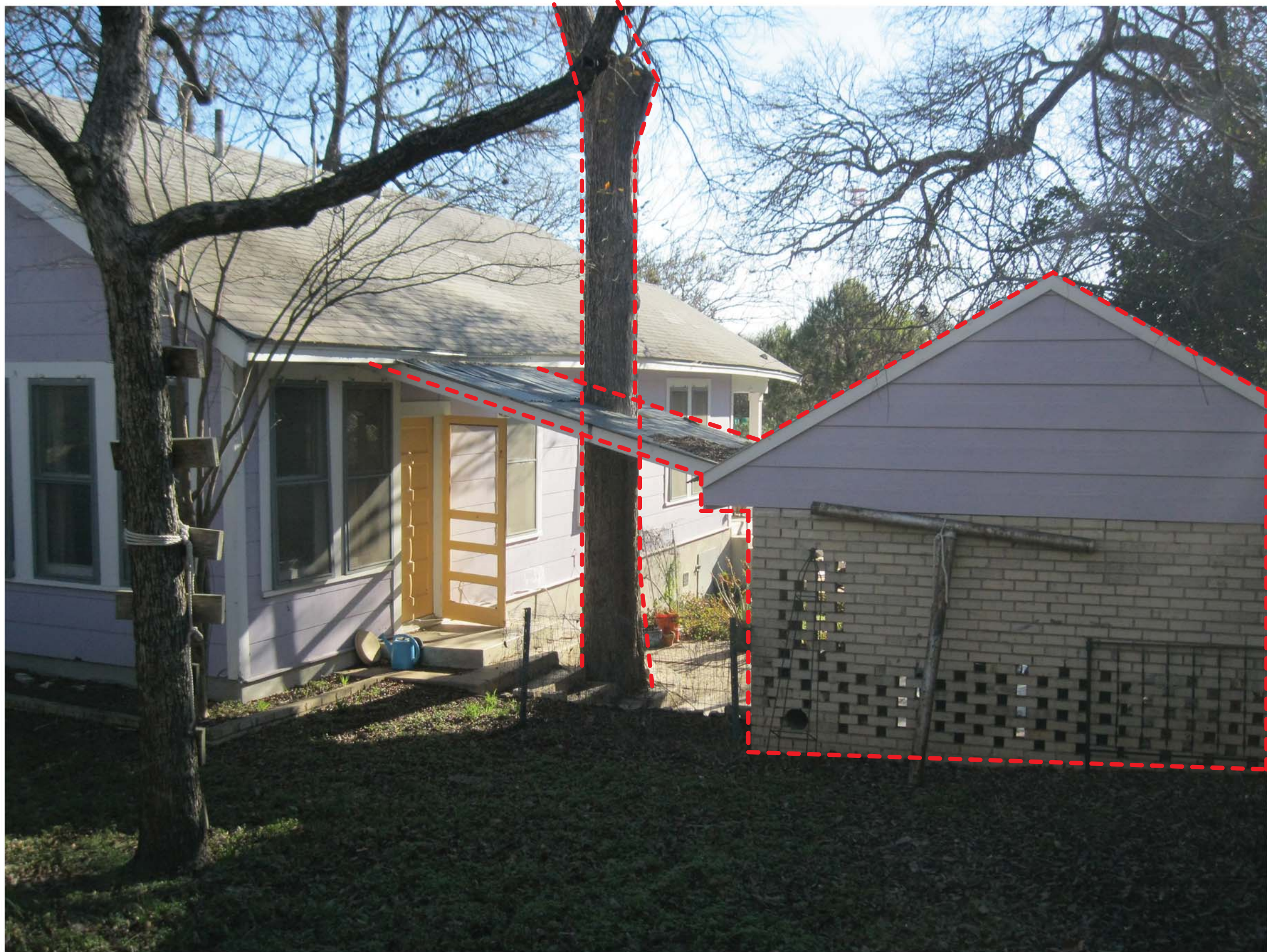
REMOVAL OF TREE, DEMOLITION OF COVERED WALKWAY, AND CARPORT
