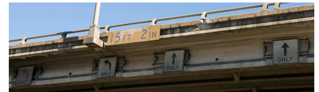
FIGURE 8 » Existing direction and instructional signage attached to interstate is extremely weathered and requires replacement.
