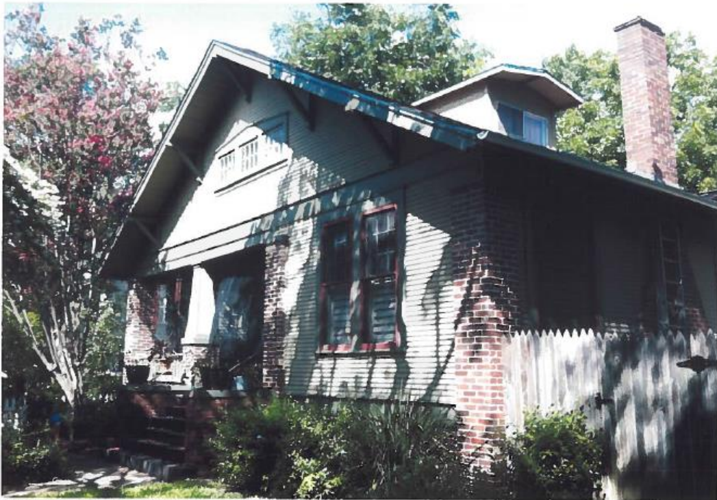
EXISTING DORMER FROM NORTH
