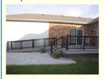
A walking surface with a running slope > 8.3% (1:12), must:
