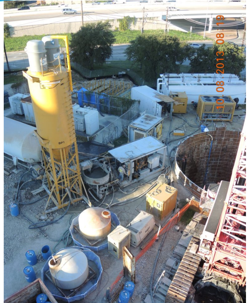
PIG Co. Grouting Operation @ Jollyville
