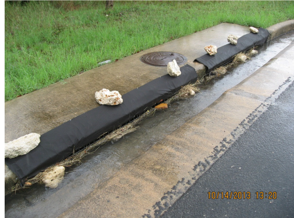
Inlet protection at Spicewood Springs Shaft Site
