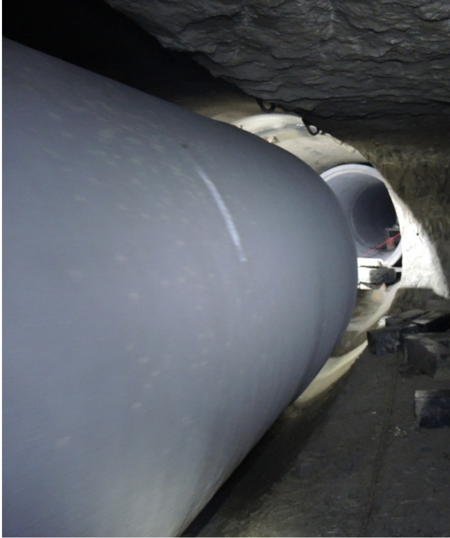
Pipe placement in tunnel
