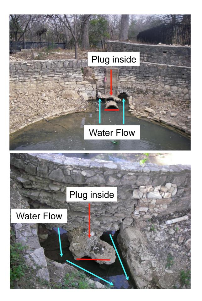
1. Enlarge outflow opening from spring pool by removing deteriorated plugged pipe.
