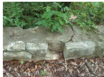
Typical cracks and missing stone
