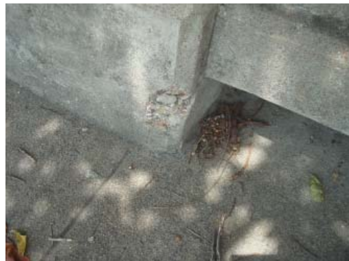
Detail of concrete spalling at guard rail
