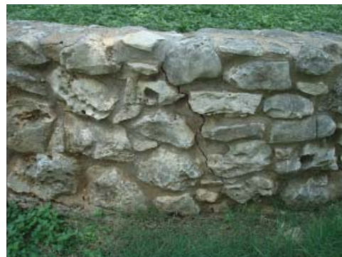
Typical cracking in wall
