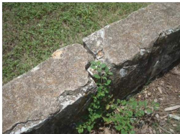
Typical through-wall crack
