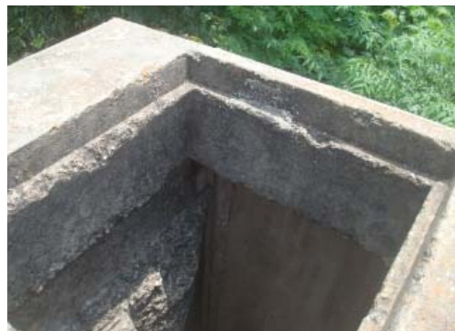
Detail of hollow pier top
