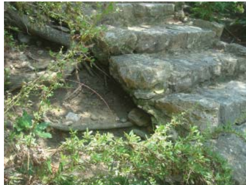
Detail of undermining on steps
