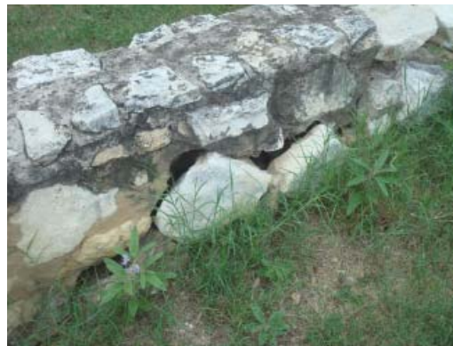
Typical cracking and stone displacement
