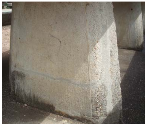
Detail at tapered, chamfered leg
