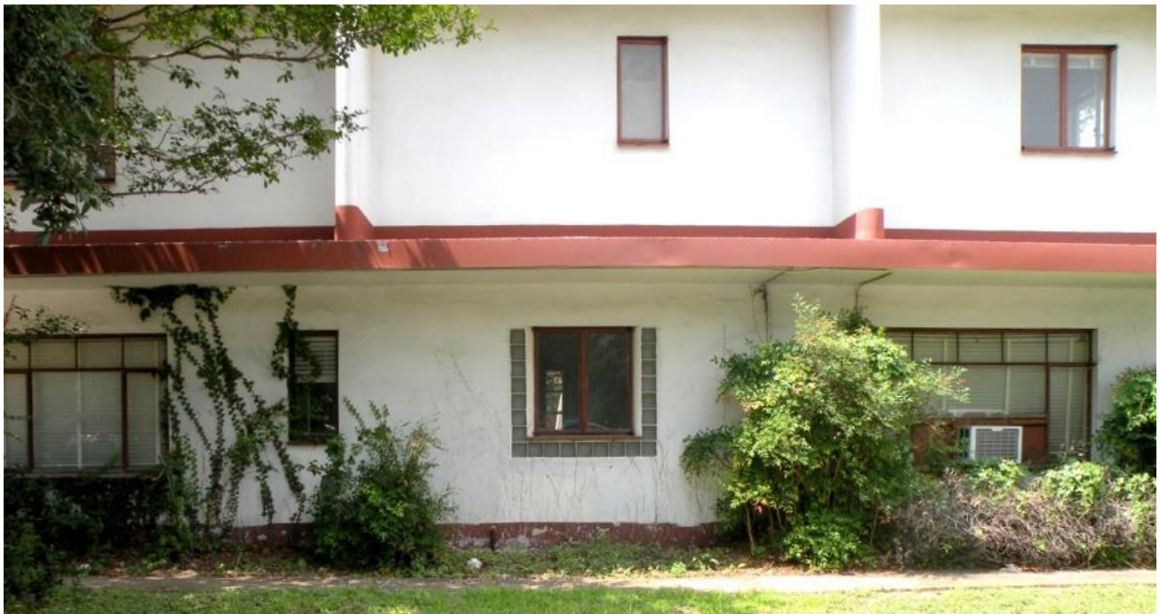
Figure 3 North elevation view of the house. There are no structurally significant cracks in the exterior load-bearing walls.
