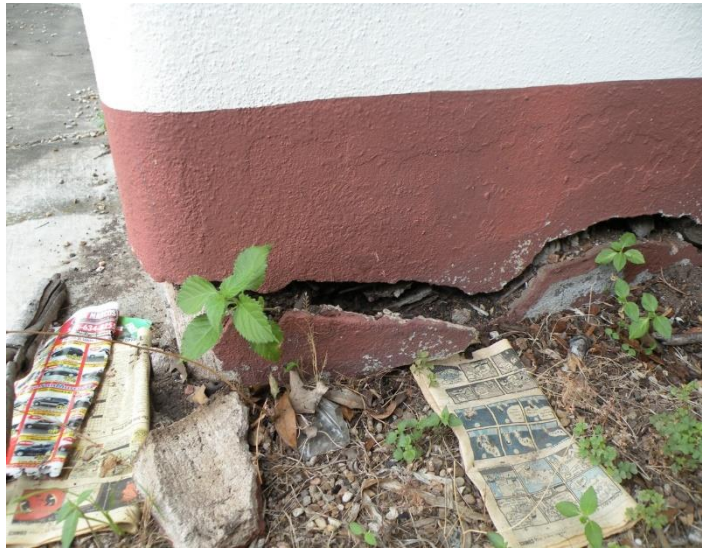
Figure 2 Distress at bottom of decorative fin is caused by rotting of the wood framing. The fins are not structural.
