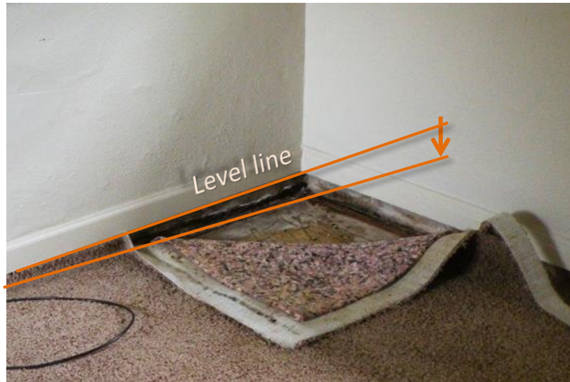
Figure 4 The interior floor slab is not supporting the exterior load-bearing walls, as seen here where the floor slab has settled independent of the walls.
