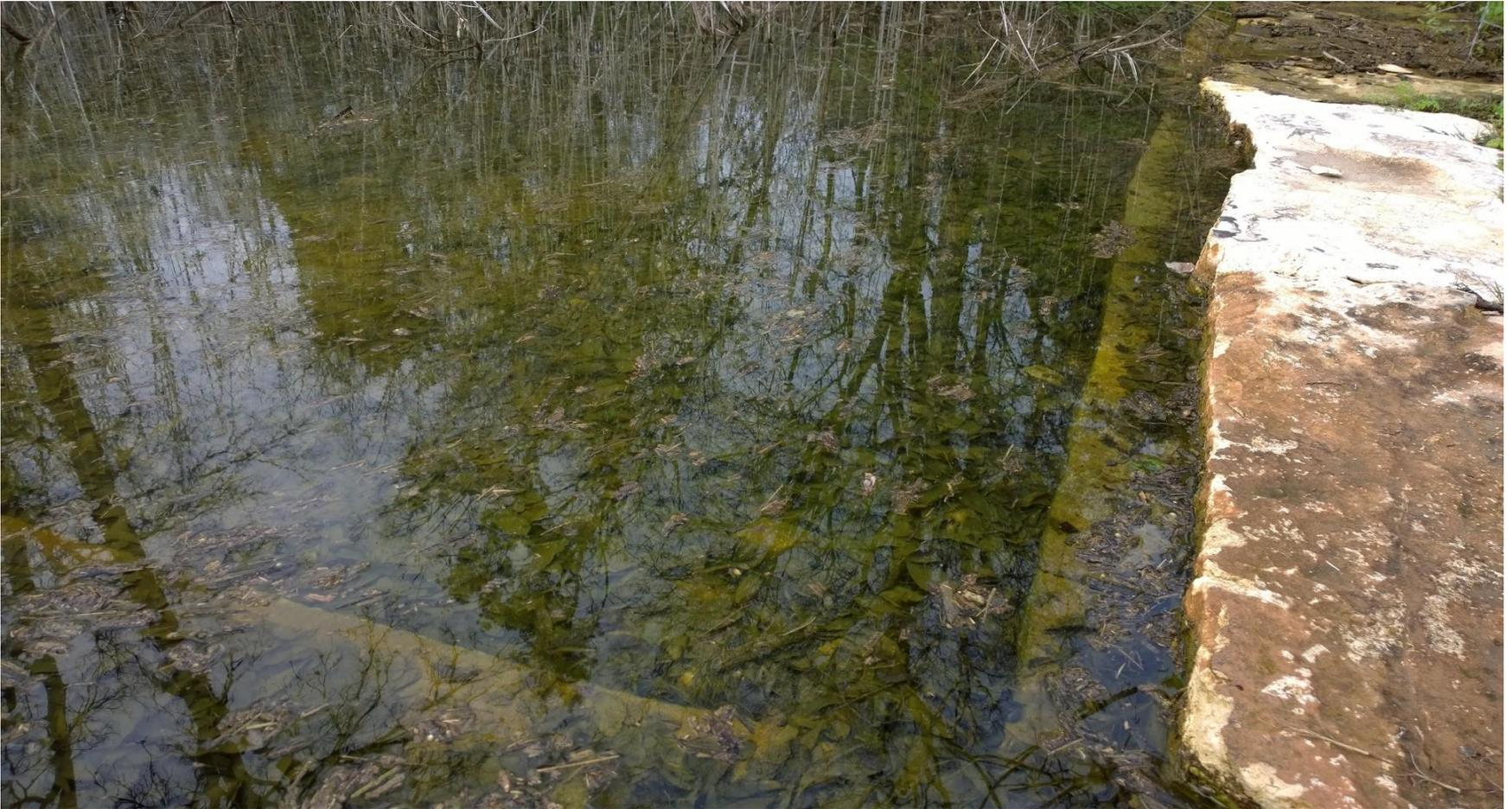
When basin is full, water appears to be seeping through natural berm and out near walkway.
