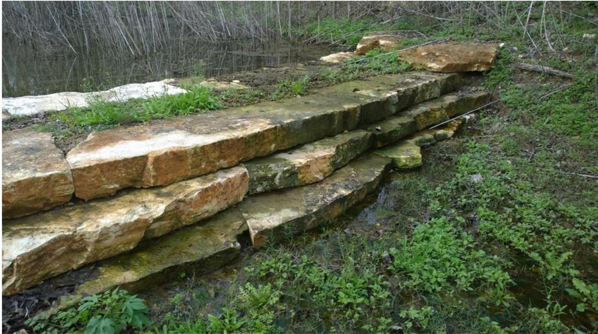
Catch basin allows sediment to settle, allowing cleaner water to flow into pool.
