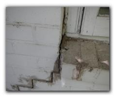
The Grade Beam at the north side of the Home (below left) near the rear corner bulges outward and has a horizontal crack due to movement.
