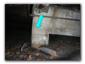
• Rotting Joists at the front wall of the north Bedroom (arrow in left photo above) are a result of leaking plumbing at the laundry hook-ups in the rear of the adjoining Breakfast Room.
