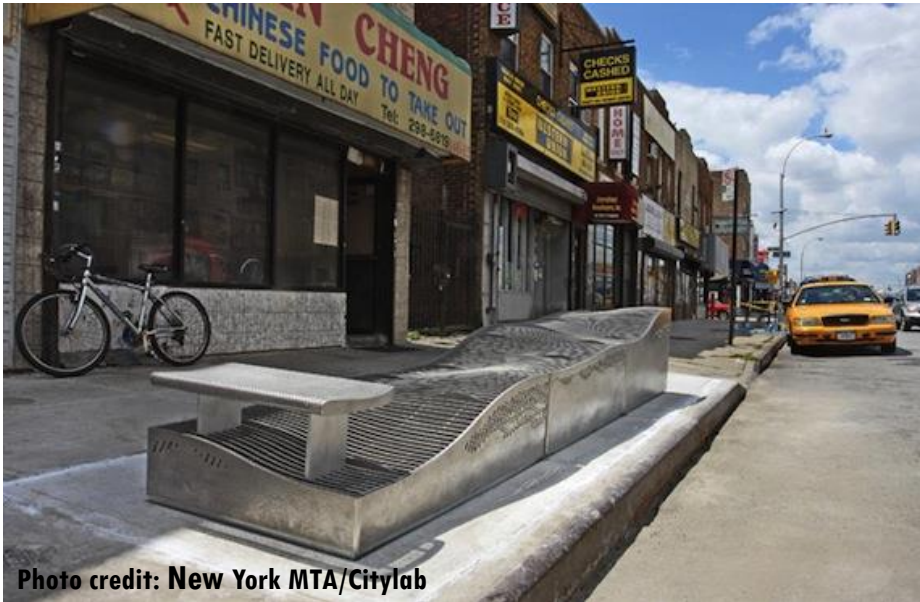
NYC design for elevated subway vents
