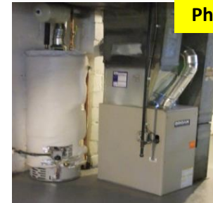
Install furnace & hot water heater
