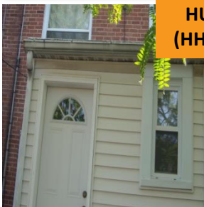
Replace broken gutters
