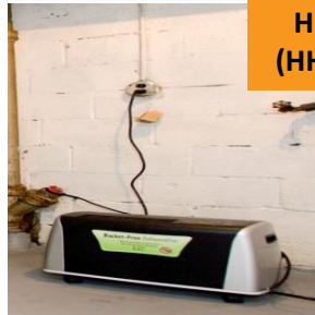
Remediate mold, install dehumidifier
