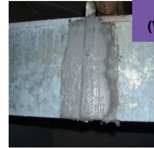
Seal ducts, blow insulation
