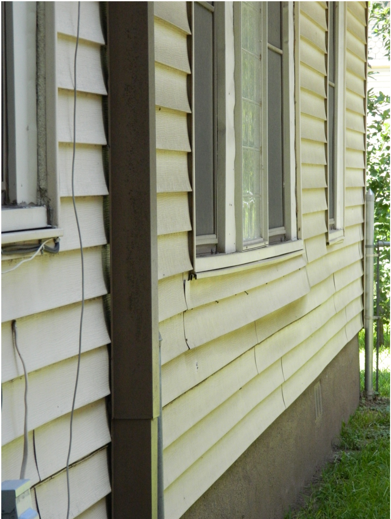
Staff photograph taken July 17, 2015 showing the condition of the vinyl siding on the house.
