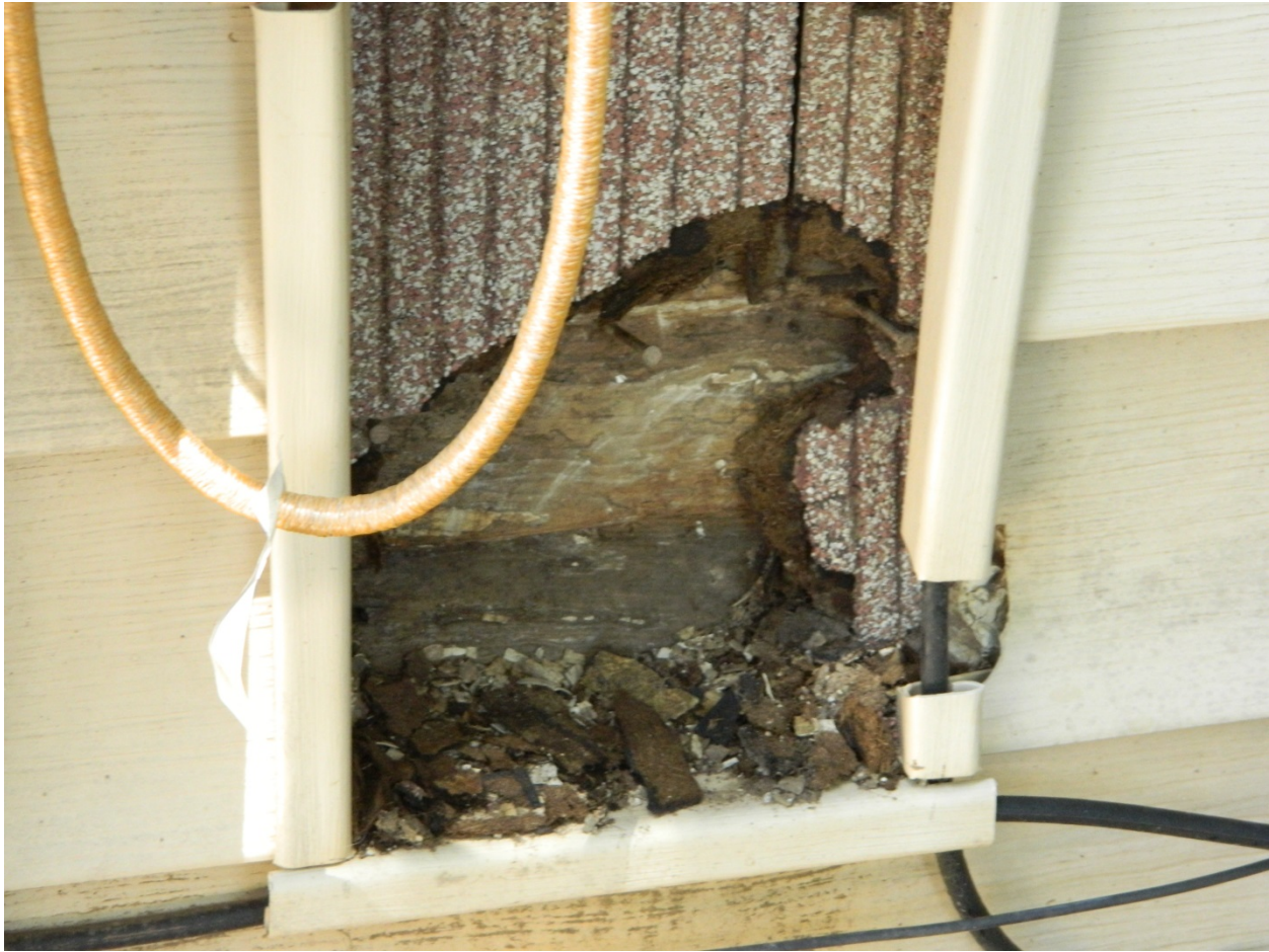
Staff photograph taken July 17, 2015 showing the vinyl siding, with asbestos siding underneath, and the condition of the original wood siding of the house.
