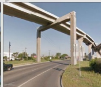
Fig. 3.5: Straddle Bent with "Longhorn" Column
