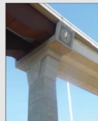
Fig. 3.3: Inverted "T" Bent, with "Longhorn" Column and Five Star Bent Cap
