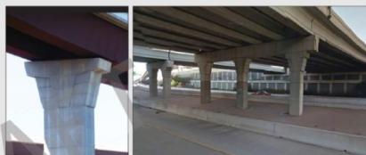
Fig. 3.1: Typical Hammerhead Bent with Rectangular "Longhorn" Columns
