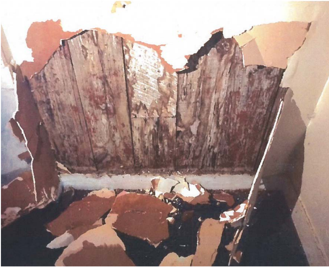
Water-damaged wood
