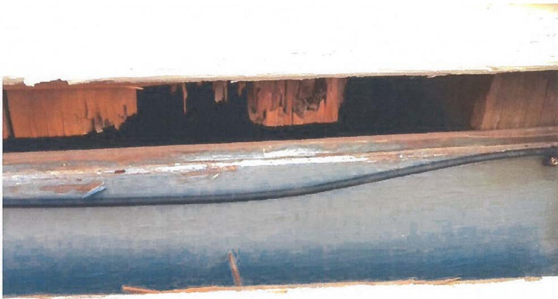
Evidence of wood rot and termite infestation at the house.
