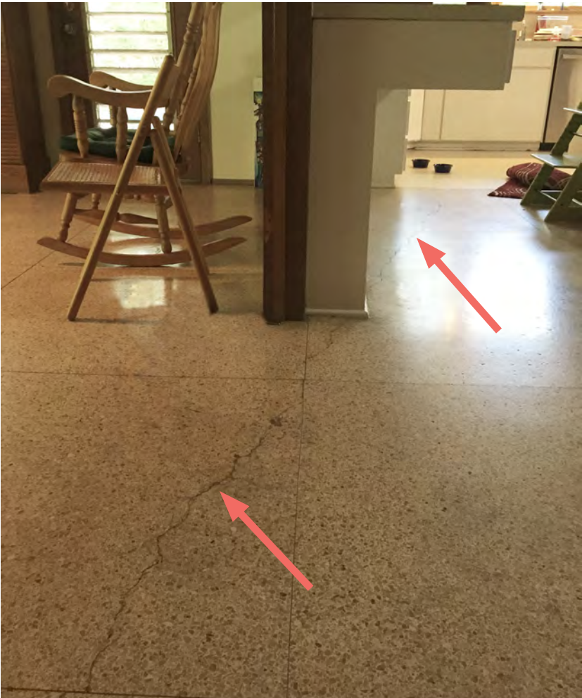
Cracked terrazzo at top of stairs into Kitchen. Any amount of foundation repair would destroy original terrazzo flooring.
