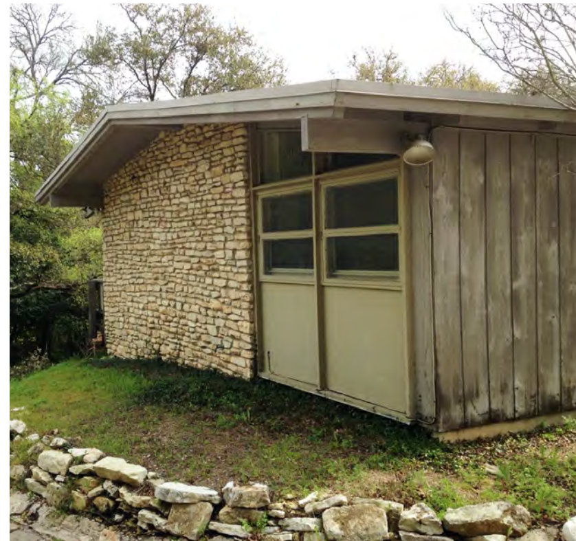
Northwest corner of Master Suite. Non energy efficient, single pane windows.
