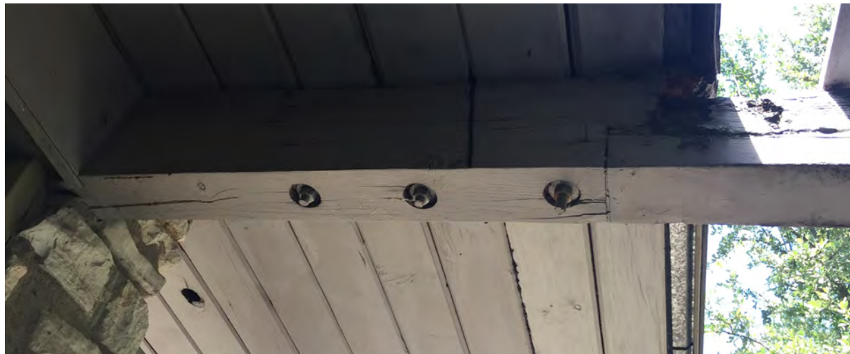
Structural roof rafters at Master Bedroom deck. Previous reinforcing for rafters is no longer sufficient. More structural repair is required at this location and other similar conditions.
