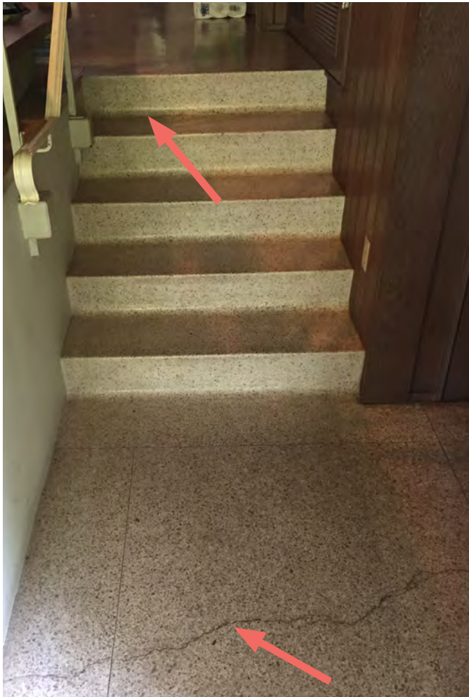
Cracked terrazzo at front door and top of stairs.
