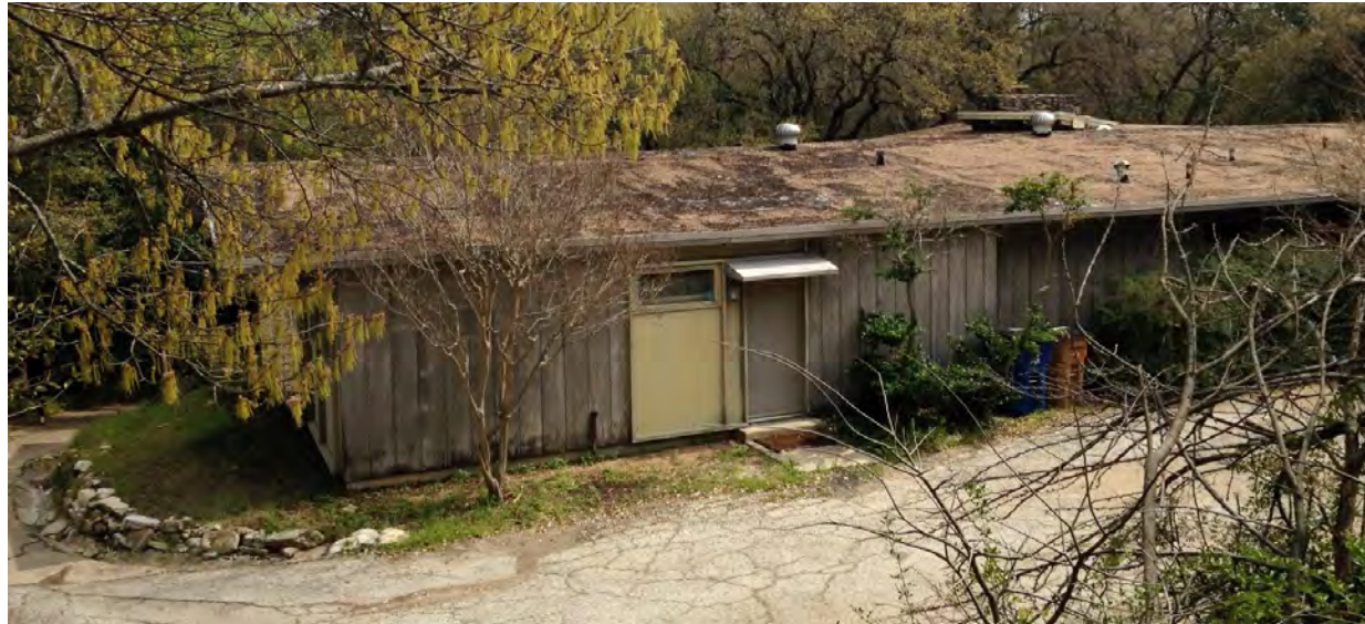
Back of bedroom wing. Roof is in poor condition, siding is rotting. No significant architectural features on this portion of the house.
