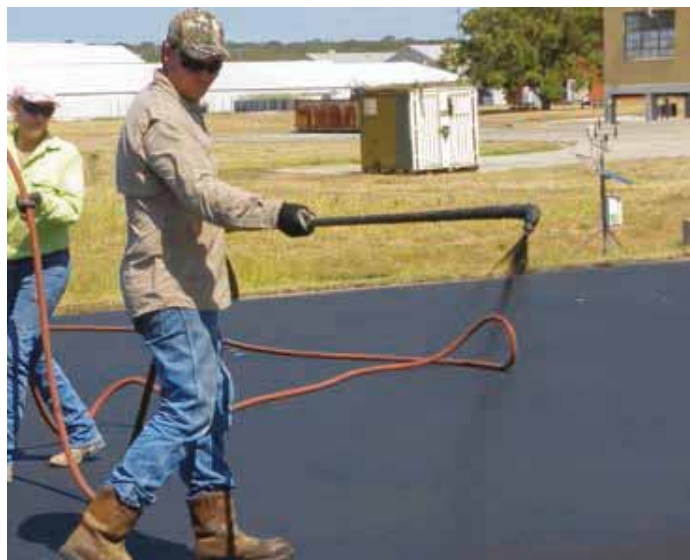
A contractor applies coal tar pavement sealers at the University of Texas, Austin for US Geological Survey research in 2011. Image by USGS
