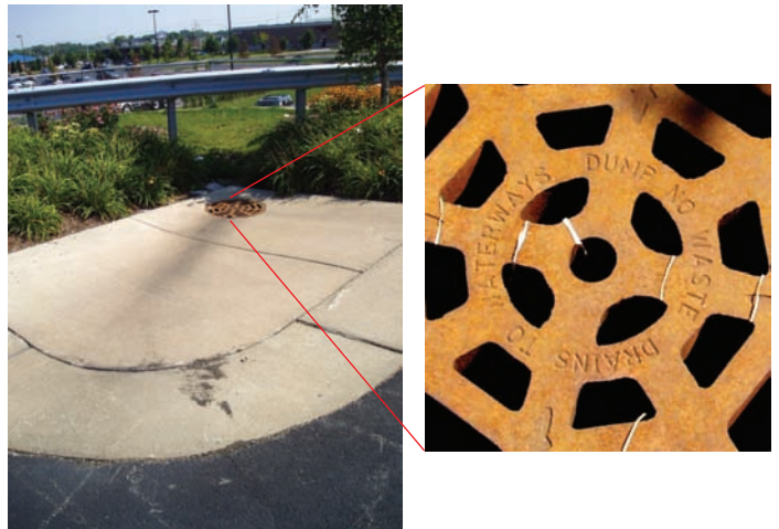
Runoff from sealcoated pavement (black surface) enters storm drains that lead to local streams. Drain grate (inset) is marked “DUMP NO WASTE” and “DRAINS TO WATERWAYS.”
